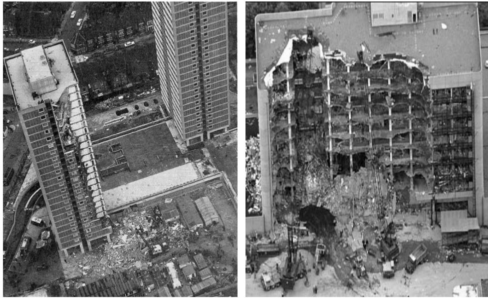
Figure 1: a) Ronan Point Apartment Building b) A. Murrah Federal Building.
