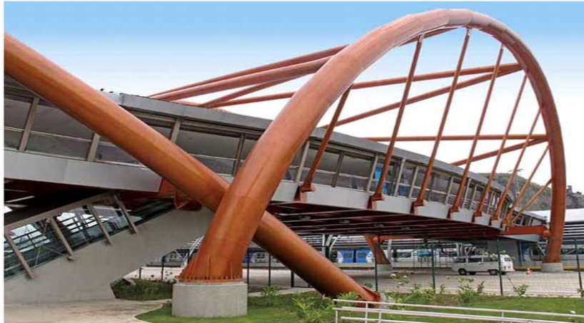
Figure 1. Example of a tubular steel pedestrian footbridge in Rio de Janeiro, Brazil.
