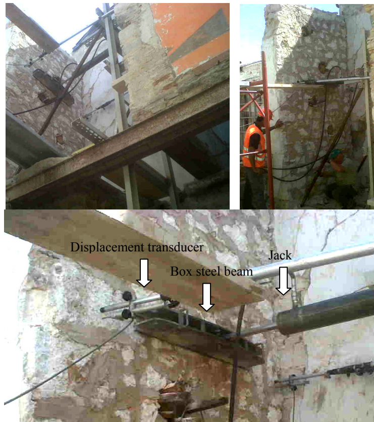
Figure 18. Details of the test set-up.
