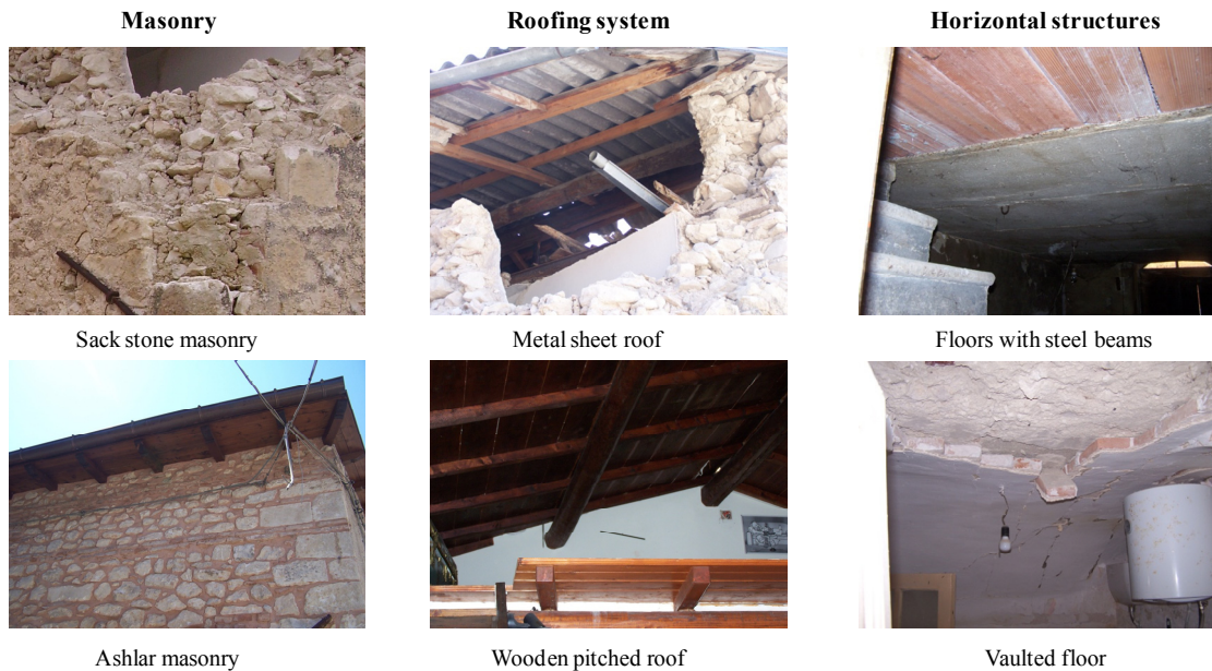
Figure 4. Main structural features of masonry aggregates of Poggio Picenze.
