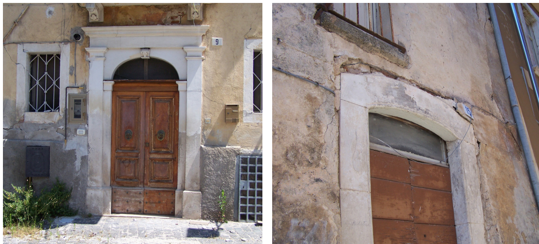
Figure 5. Architectural cornices made of the so-called white stone of Poggio Picenze.
