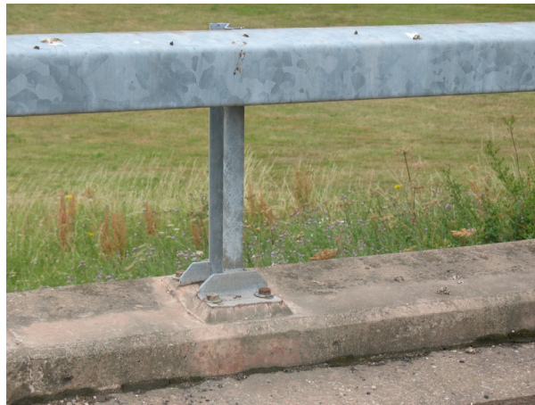
Figure 2: Road barrier behind a kerb
