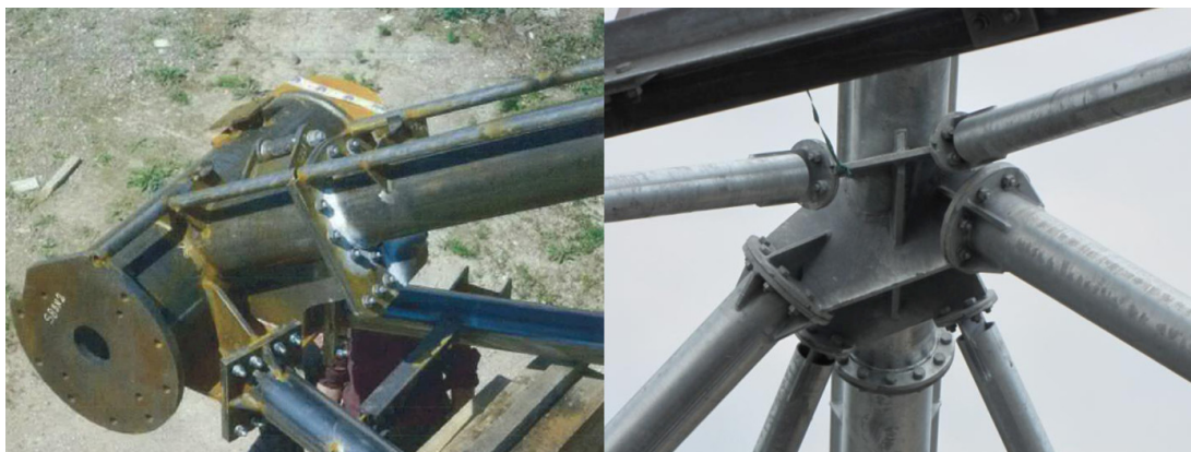
Figure 4: joint with 3 converging structural members (left) and 6 structural members converging at the chord (right)
