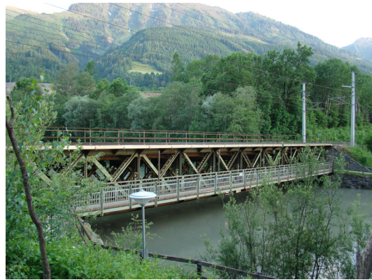
Figure 8: Salzacherbrücke (A) constr. 1907, line Salzburg - Wörgl, span 40 m
