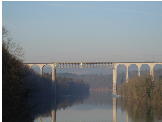
Figure 7: Eglisauer Bridge (Switzerland), Constructed 1895-97, line Eglisau – Hüntwangen, span of steel truss 90 m
