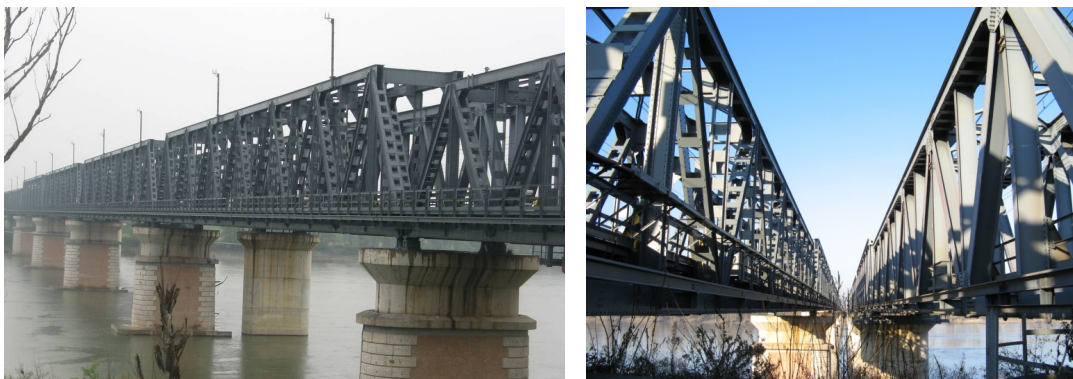
Figure 1. The Pontelagoscuro viaduct on the Po river.
