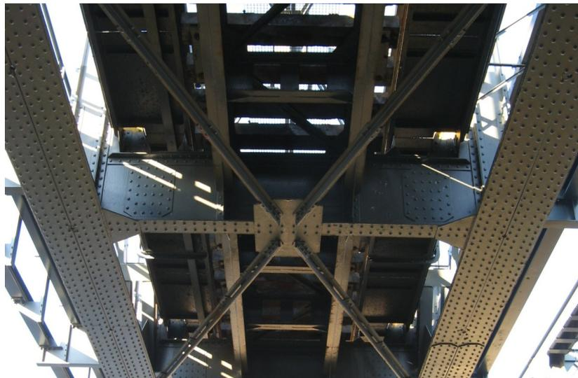
Figure 3. Details of lower bracings, floor-beams and stringers.
