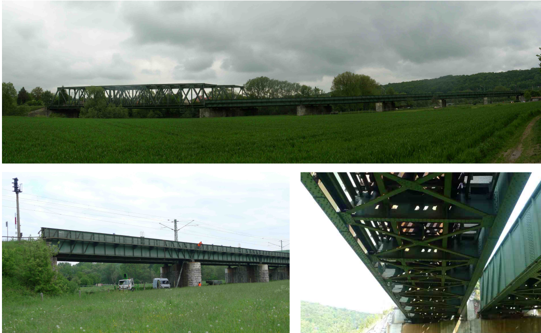
Figure 1. Saalebrücke: complete aspect (top), considered plate girder span (bottom left), view from underneath the bridge (bottom right).
