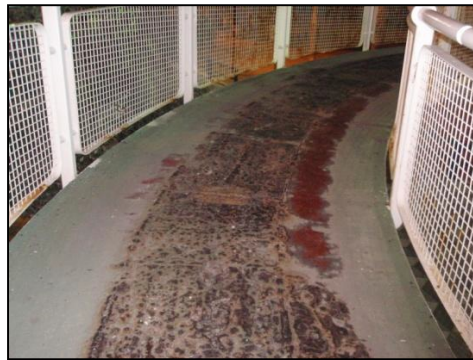
Figure 2: Degradation phenomena due to corrosion from chloride.
